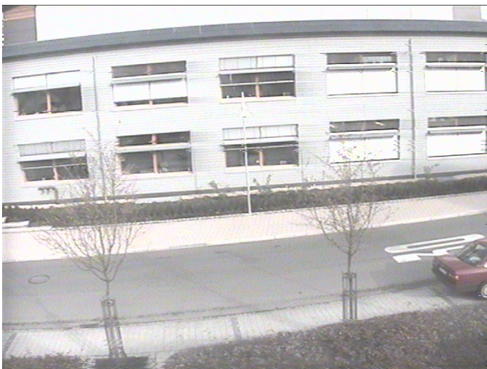
Fig. A.6.1-3: Example picture of the monitored facade with the 10 offices.
