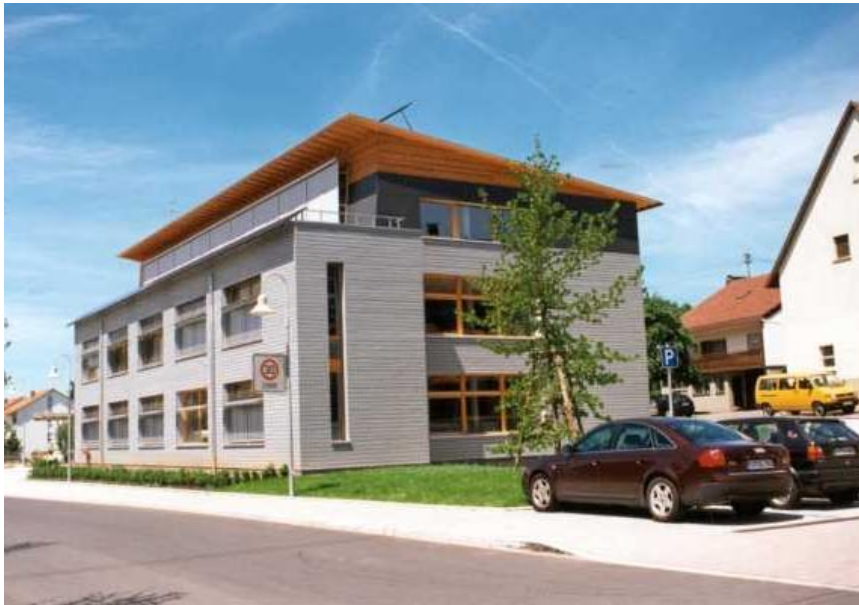
Fig. 6-4: Photo of the monitored Lamparter building 54 . (architects: Meier-Weinbrenner-Single, Nürtingen, Germany, Photo © K. Voss)
