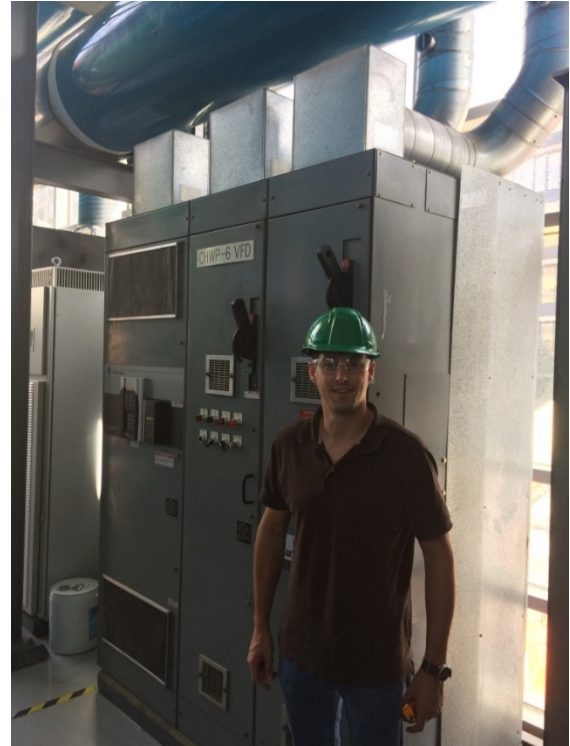
Fig. 16: Size comparison with 500 hp VFD
