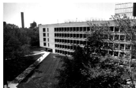
Dreyfus Chemistry Building, constructed 1960s, renovated 2000s.
