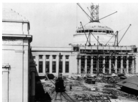
Construction of the original Cambridge campus, 1910s.
