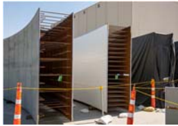
Vogtle Unit 3 shield building wall panels, May 2014
