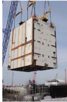
CA20 being set in place by heavy crane
