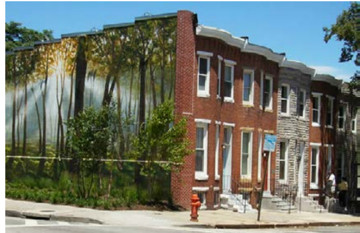
Renovated housing for Martha's Place with mural and memorial garden.
