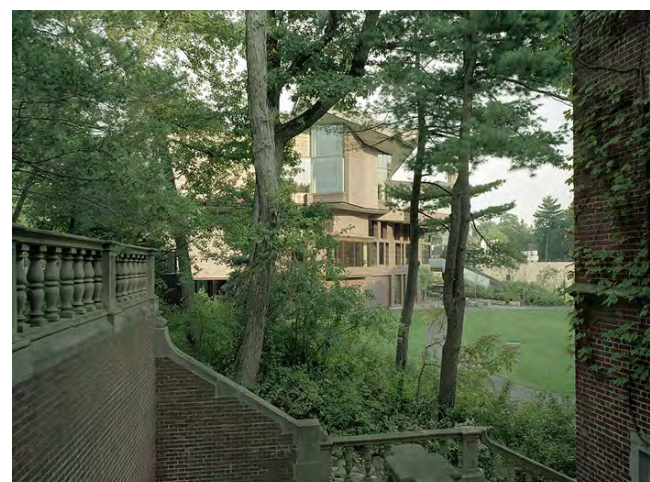
(1d) Portal at Wellesley College, Wellesly MA
