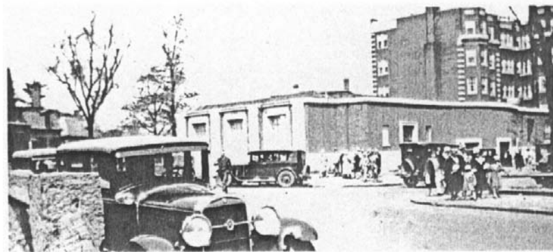
Figure 1. The first phase of construction terminated at the belt course (First Church, 1996).
