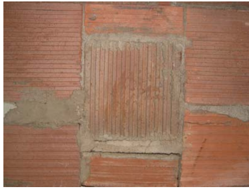
Figure 10. Corrugated surface of the structural and hollow terra cotta tiles.
