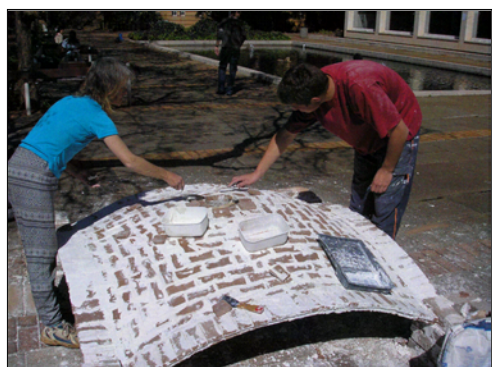
Tile vault has little formwork
