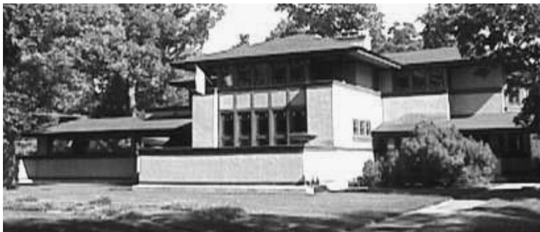
Figure 11. Prairie house: exterior of Wright's Willits house, Highland Park, Illinois (1901)
