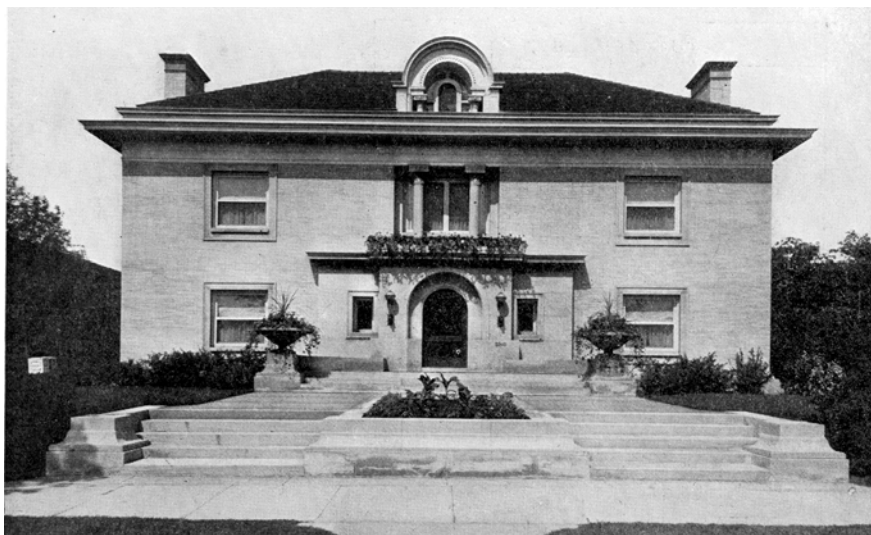
Figure 14. Non-Prairie house: George Maher's Colvin house, Chicago, Illinois (1915)
