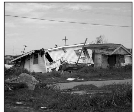
Destruction rendered by Hurricane Katrina
