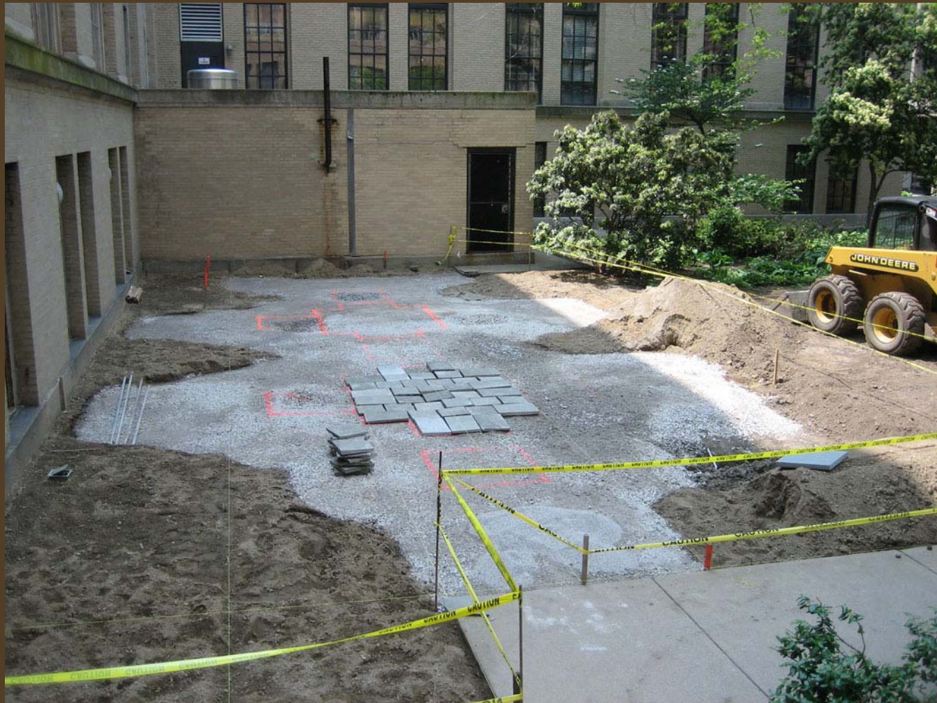
Recycled bluestone pavers from demolished Dibner Garden
