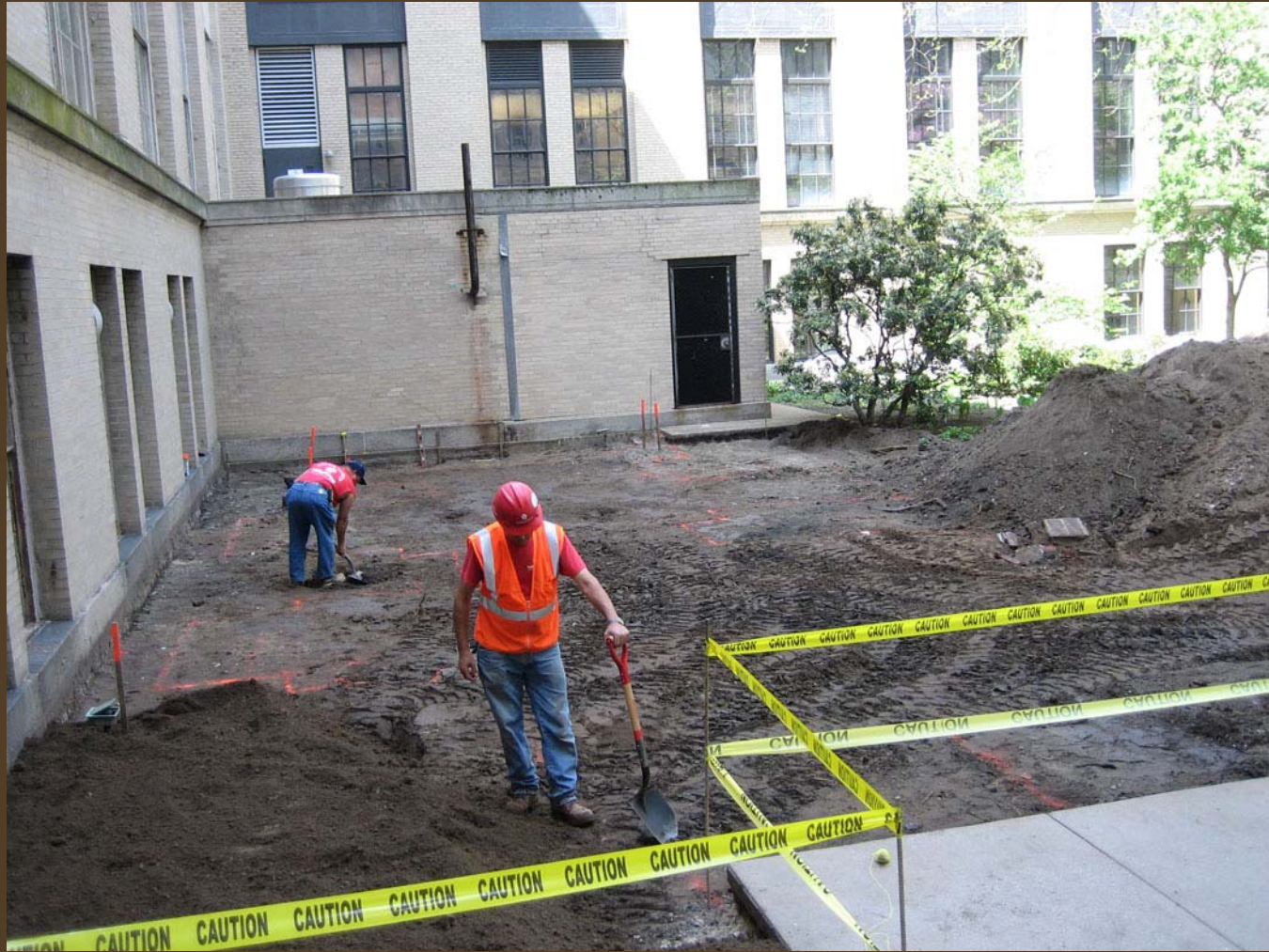
Valley Crest starts construction
