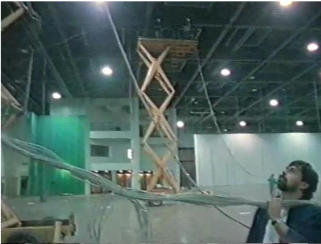
Figure 6: Screen grab of the construction of the Interop trade show's INTEROPnet (or ShowNet). The routing and bridging equipment used to construct the show network was estimated to have been as much as a major corporation would use to supply offices in fifteen or twenty cities.<sup>34</sup>
