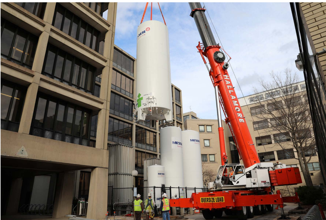
Added 13,000-gallon N 2 tank and upgraded vaporizer.
