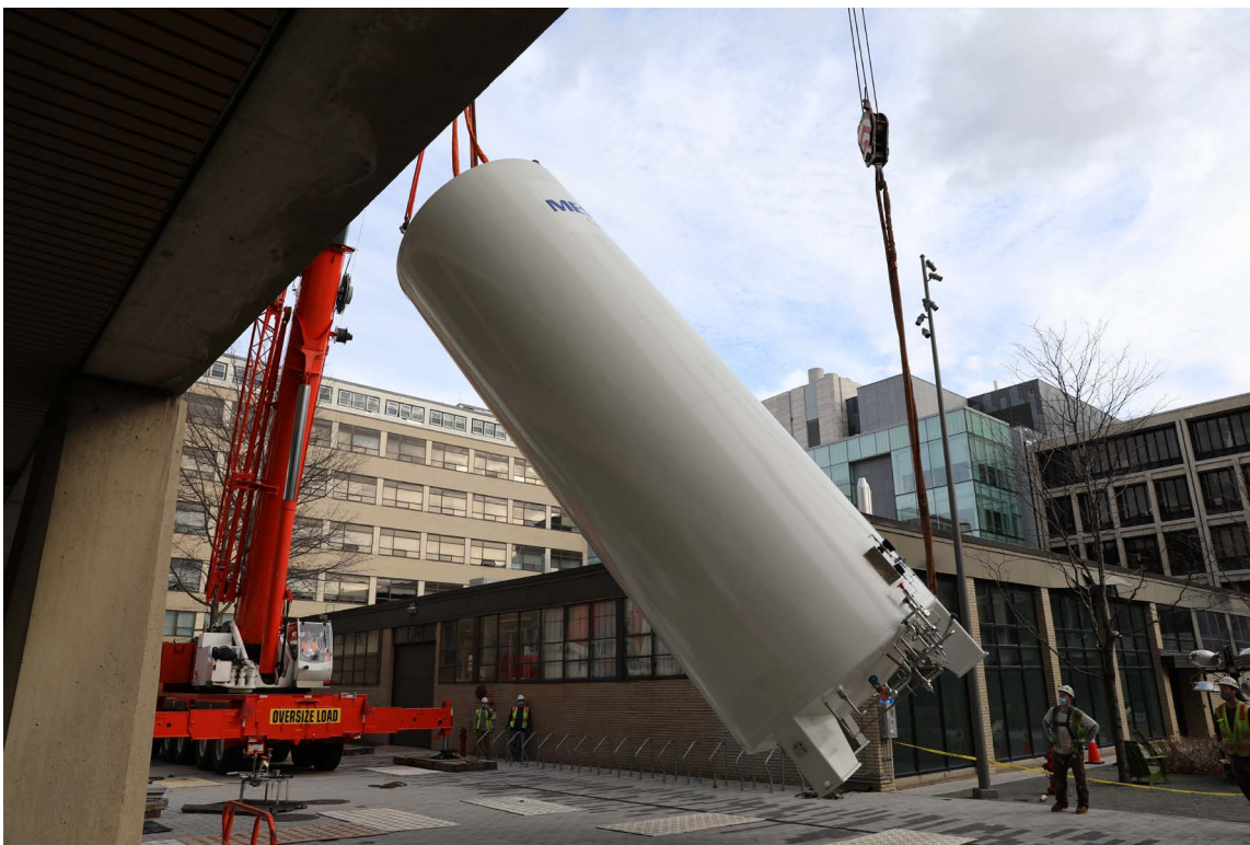
Replacing O 2 tank.
