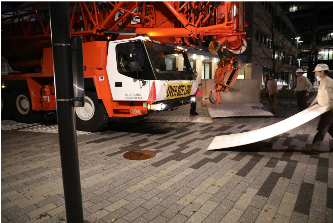
4:00 am start time protecting cobblestones.
