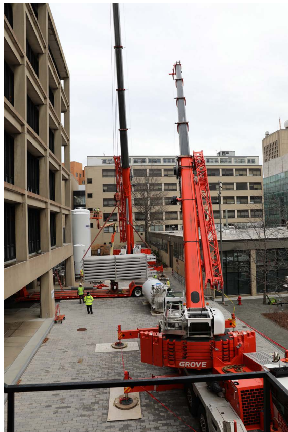
240-ton lead crane and 175-ton helper crane.
