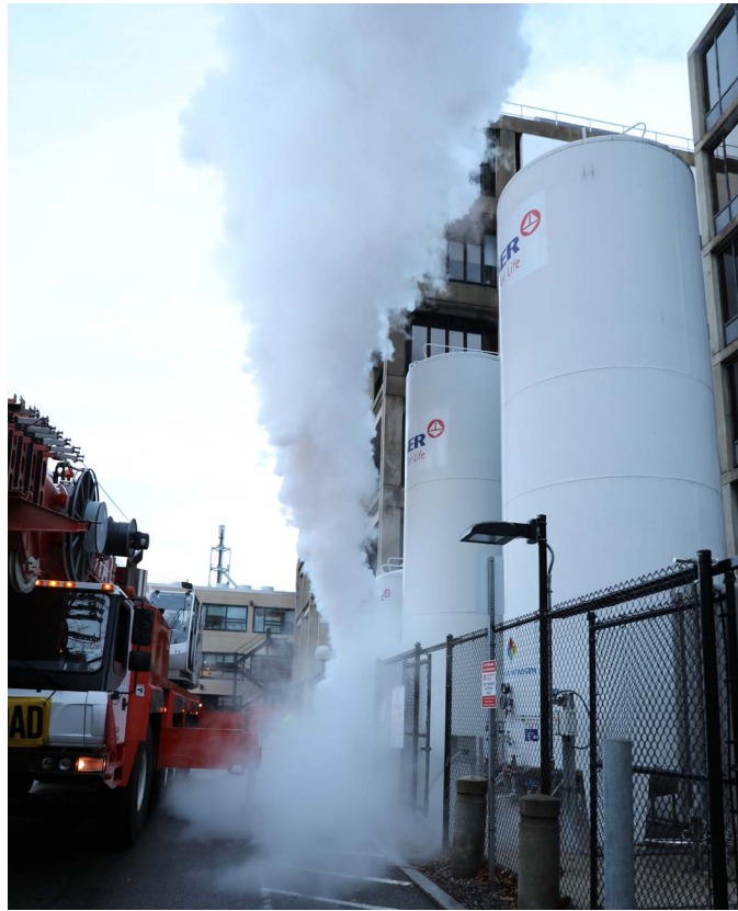
Controlled O 2 depressurization before tank removal.
