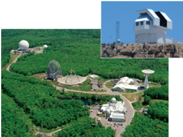
Figure 9. The tactical space situational awareness initiative is utilizing the Space Surveillance Telescope (above, inset) and the Haystack Ultrawideband Satellite Imaging Radar and Millstone Hill Radar (above) to demonstrate data fusion and sensor handoff approaches for improving the timeliness of the US Space Surveillance Network, with the objective of achieving tactical command-and-control responsiveness.
