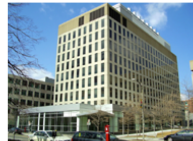
Figure 7. ISN headquarters and labs occupy the fourth and fifth floors of 500 Technology Square (NE47) in Cambridge, MA.
