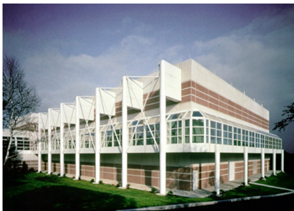
Figure 7. Microelectronics Laboratory. Upgrades in 2010–2011 provide the capability for production-class sub-90-nm processing on 200-mm wafers.
