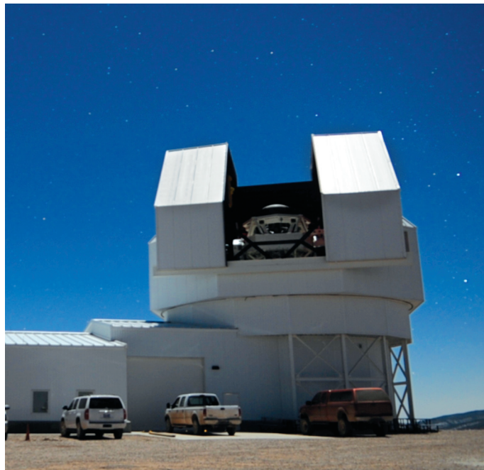
Figure 3. The Space Surveillance Telescope in its enclosure on North Oscura Peak in New Mexico.
