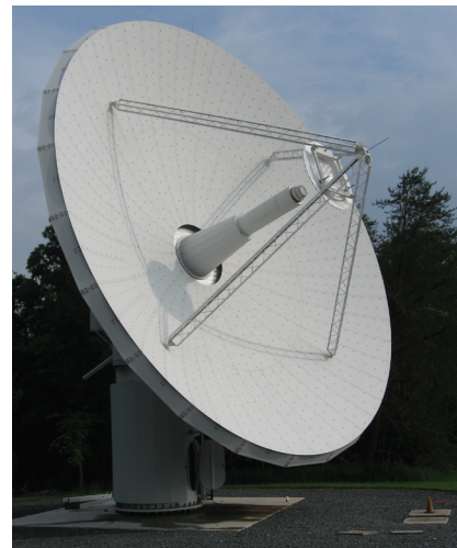
Figure 3. The new 12-meter antenna in Greenbelt, MD, forming part of the new VLBI2010 geodesy system being developed at Haystack.
