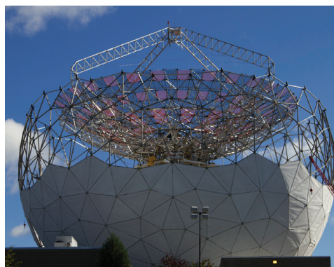
Figure 2. The appearance of the Haystack 37m telescope in mid-September 2010. The old reflector had been removed, and the backup structure and quadrupod of the new reflector had been installed. Following this, the radome cap was reattached, the radome panels were replaced, and the reflecting surface panels were then attached to the backup structure in a weatherproof environment.
