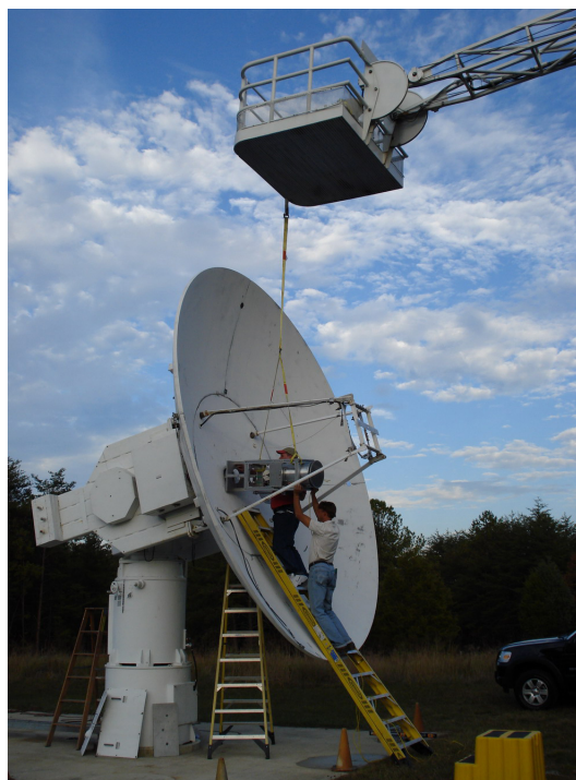
Figure 4. A prototype broadband frontend system being installed on the 5 m GGAO antenna at NASA GSFC. This advanced system is part of a program whose goal is to make global geodetic-VLBI measurements with a precision of 1 mm.
