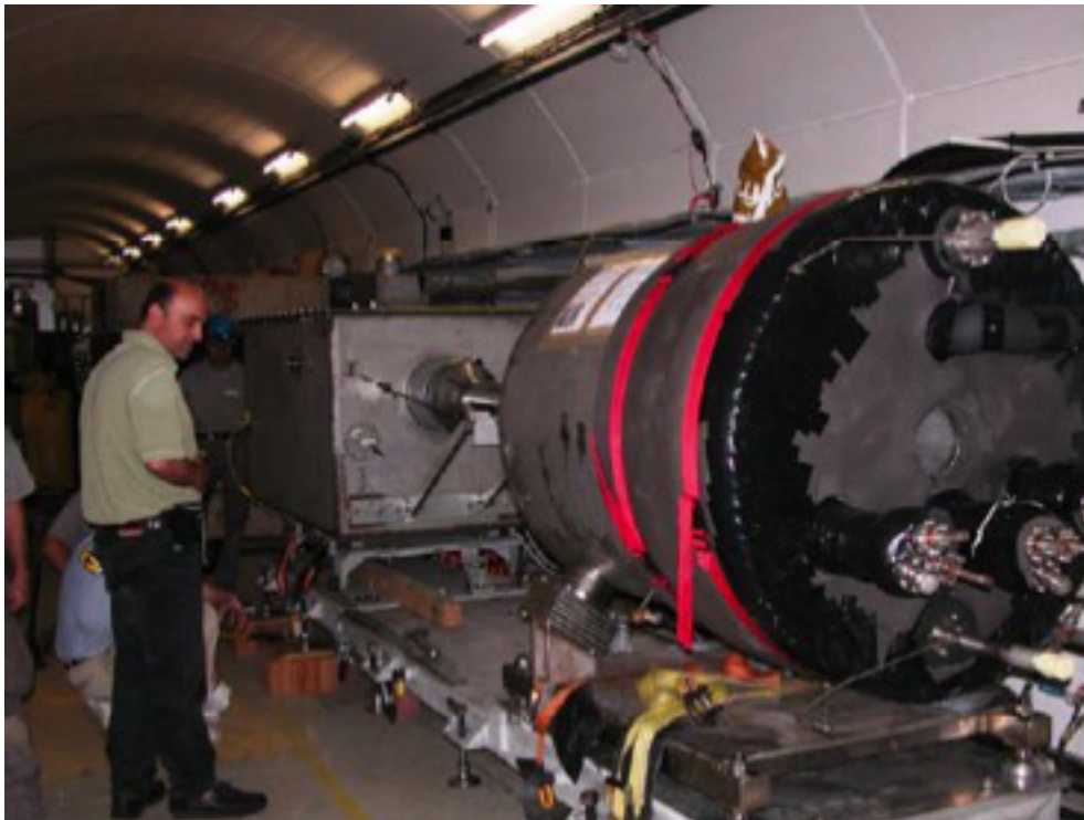
Figure 7. MERIT magnet and mercury jet target being installed at CERN.
