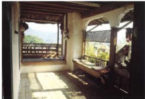
Image 3.5. Open veranda in front of a room of a Menteşe Mountains' house, sunny in winter (above) and shaded in summer (down) (Aran, 2000: 98-99).
